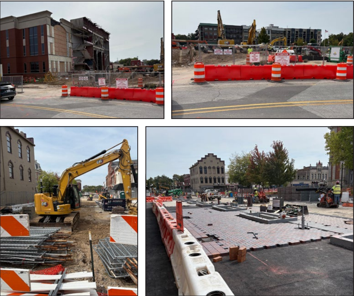
Reporter photos The expansion project on the west side of the Hamilton County Government and Judicial Center is well underway. The $70 million expansion will add 133,000 square feet to the Judicial Center, including seven new courtrooms, upgraded security, and more public space. The project is expected to be complete at some point in 2028.
