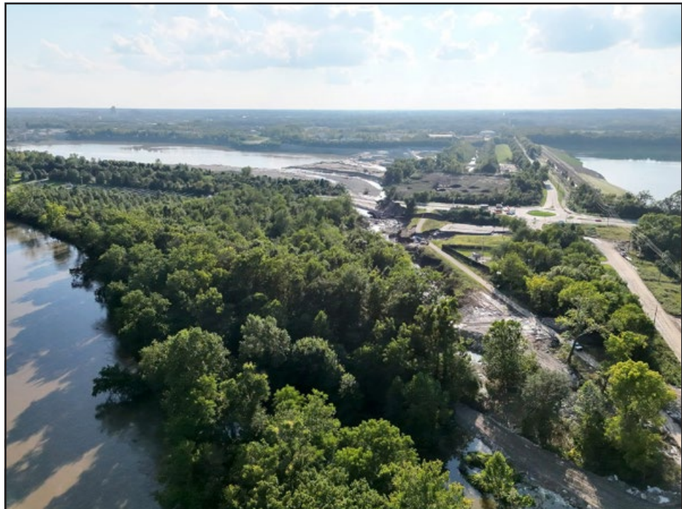
The work is ongoing following historic flooding in Hamilton County. Here, you can see the area near the collapsed bridge and the Martin Marietta quarry in Carmel. This aerial photograph is oriented west at the intersection of Hazel Dell Parkway and 106th Street.
