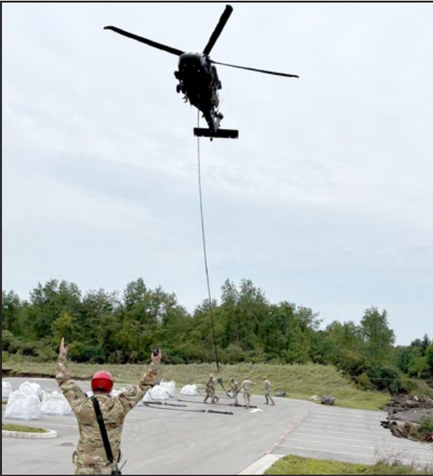
Photos provided by City of Carmel In addition to all the manpower that went into construction the two temporary dams, the Indiana National Guard deployed two UH-60 Blackhawk helicopter crews to move 73 sandbags weighing 2,000 pounds each to build the secondary dam.
