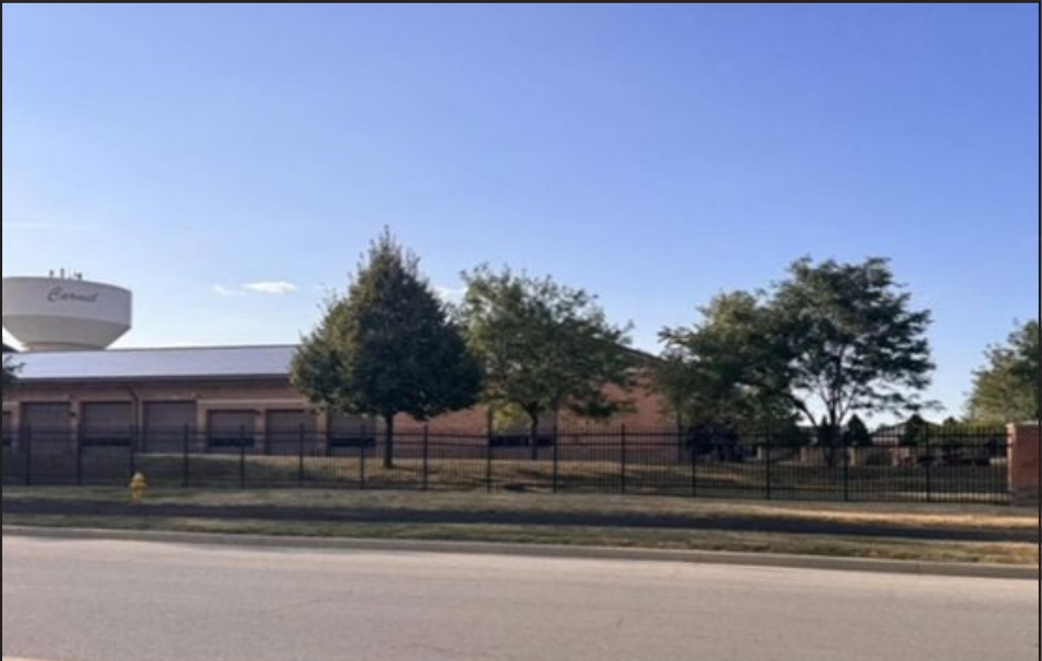
Photo provided by City of Carmel This is the site for the new fire station is at the water distribution facility on Carmel's west side.
