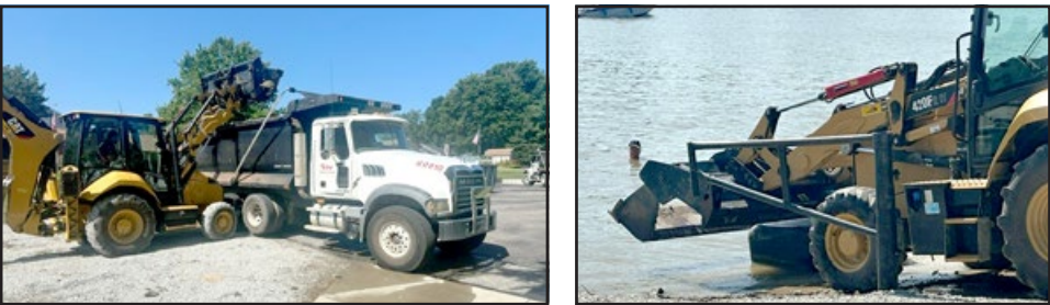
The Town of Cicero provided a front-end loader and operator to fill the dumpster and trucks.
