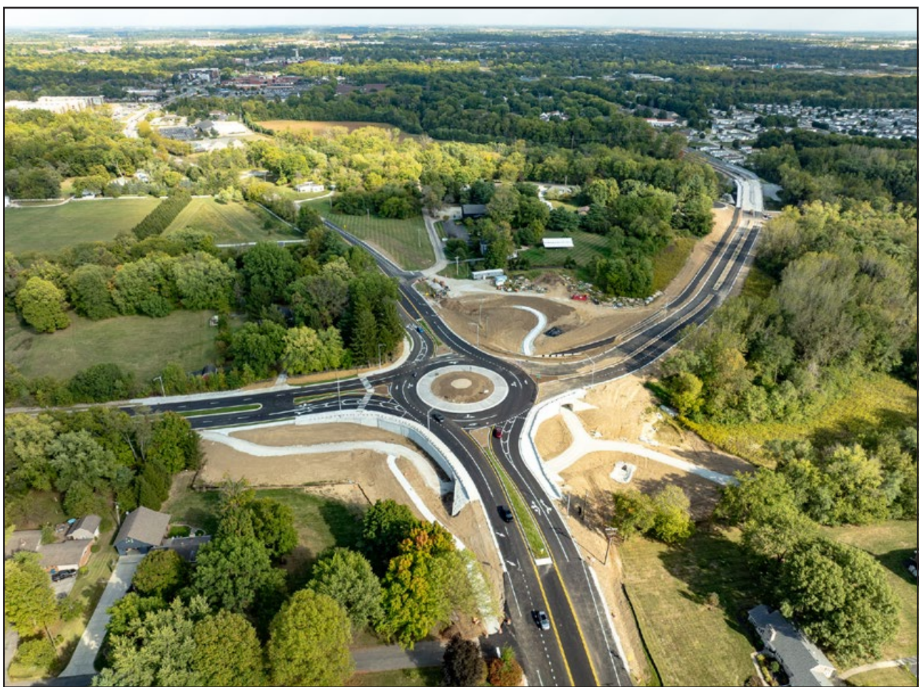
The new roundabout at State Road 32 and Hague Road serves as the west-end connection point with the new Pleasant Street. This photo looks toward the southeast, with Downtown Noblesville in the upper-left portion of the picture.
