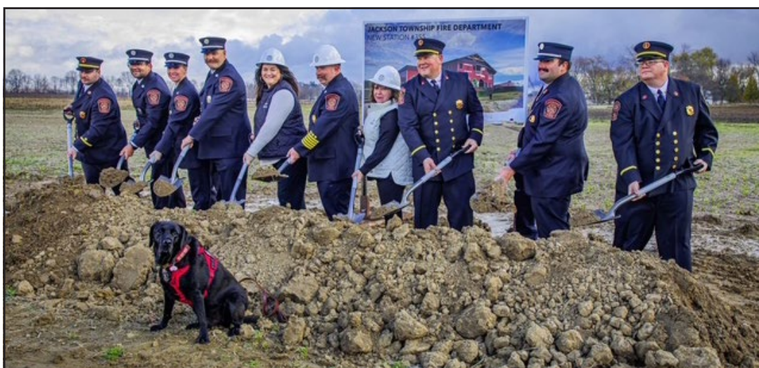
Thanks to Beck's Hybrids, Jackson Township will have a new, high-class fire station, community center, and township offices.
