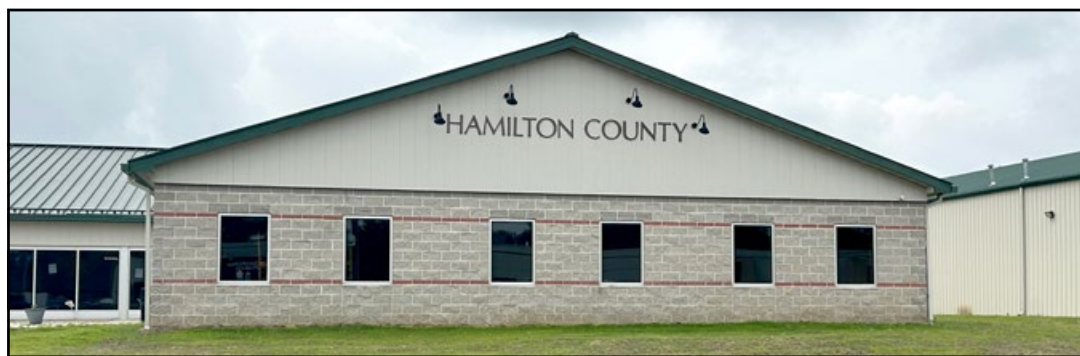
The 12,000 square-foot building will eventually house the county's Hazardous Waste Department, Soil and Water District, and Weights and Measures offices.
