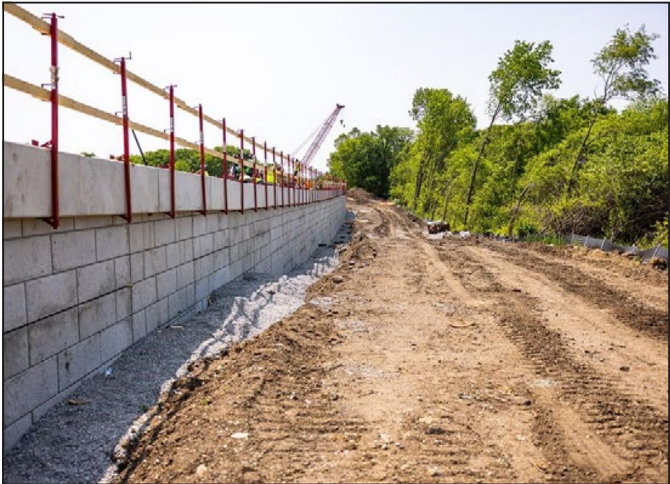
Photo provided by American Structurepoint Retaining walls are being installed for the new bridge over the White River.
