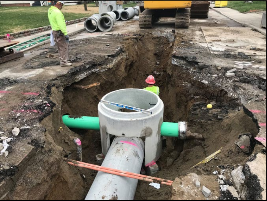
Photo provided The City of Noblesville has announced its Long Term Control Plan Phase 5 work wrapped up on 16th Street on Wednesday. The work included installing a conflict structure manhole. According to city officials, there are various utilities that conflict in this area. Crews have begun saw cutting the asphalt on 14th Street and will start construction on Thursday to install the new storm pipe from Conner Street to Maple Avenue. City officials said that because of the narrow complexity of 14th Street, it may need to be closed through the weekend and into next week.
