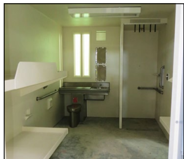
Reporter photos by Jeff Jellison (Left) Individual prefabricated jail cells weighing 17,000 pounds are stacked on top of each other with a cement catwalk to be constructed for the upper floor. (Right) New jail cells will have their own shower stalls. The expansion project's design will allow maintenance workers to access each individual cell's utilities from a hallway located behind the cells, eliminating the need for maintenance staff to enter an area containing inmates.
