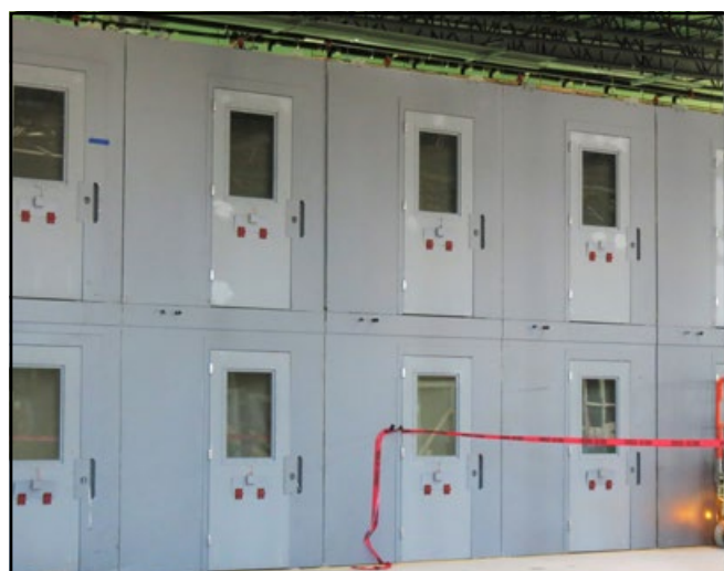
Reporter photos by Jeff Jellison (Left) Individual prefabricated jail cells weighing 17,000 pounds are stacked on top of each other with a cement catwalk to be constructed for the upper floor. (Right) New jail cells will have their own shower stalls. The expansion project's design will allow maintenance workers to access each individual cell's utilities from a hallway located behind the cells, eliminating the need for maintenance staff to enter an area containing inmates.
